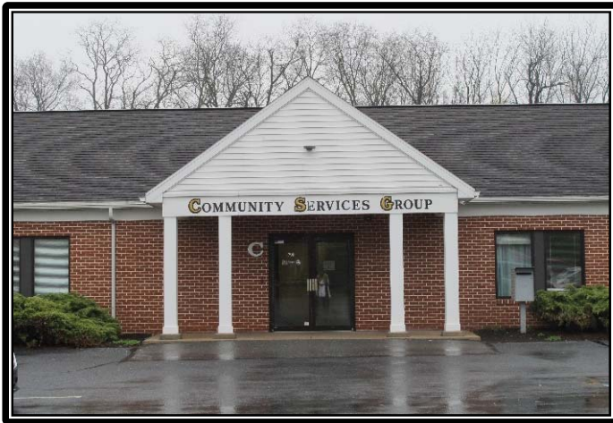
Main Lobby Entrance
