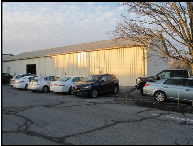
Building Front – North Lane
